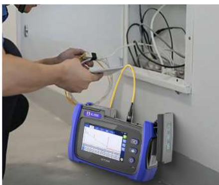
Broadband construction in residential area
