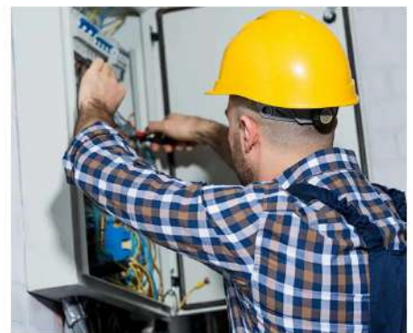
Installation and maintenance works
